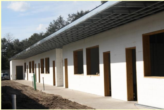
Well under way!
